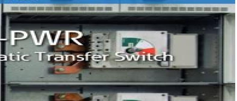
The Eaton Automatic Transfer Switch (ATS-PWR) monitors the incoming AC mains supply (1 or 3 phases) for under voltage, over voltage, under frequency, over frequency and voltage unbalance. In the case of any mains supply disproportion it will send a remote start command to the generating set and make change over for both generator and mains contactors.
