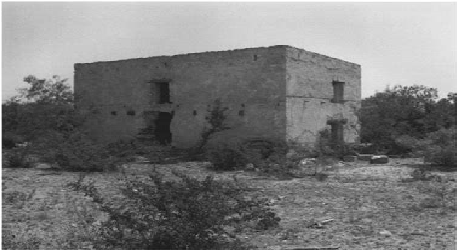
Two-story Spanish colonial main house. This casa mayor is made of sillares (caliche blocks), quarried from beneath the topsoil. Courtesy John E. Conner Museum.
