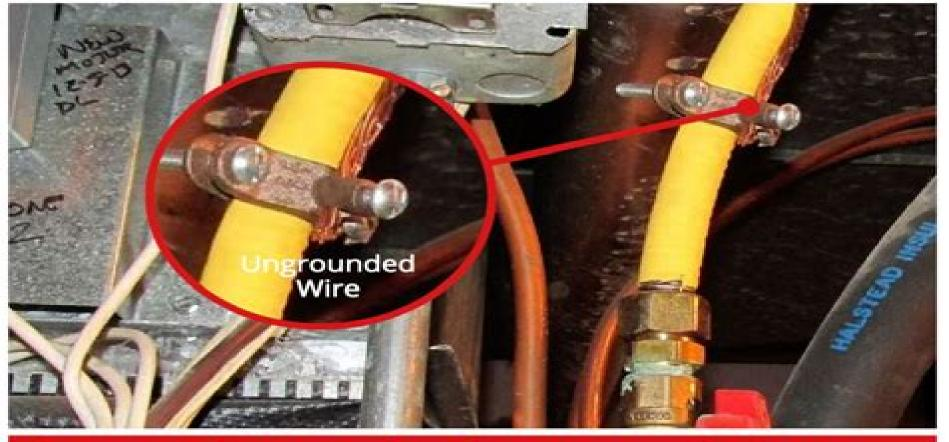
The ground wire in this photo is attached to a CSST gas line, which is improper. As a result, any outlets depending on this ground will remain ungrounded, which can lead to electrical shock, fires, and/or the failure of any equipment plugged into them.
